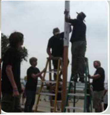
Installation of a Ventura, CA SLAP pole
