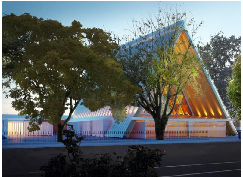
At night, the light from inside the Diocese of Christchurch’s Transitional Cathedral will make the building appear to glow through the polycarbonate roof from the gaps between the cardboard tubes. Photo/Christchurch Cathedral
